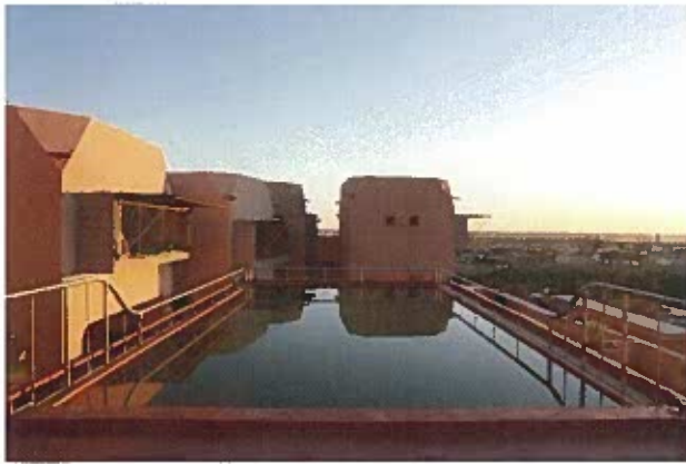
The warm hues of the walls were created with lime and natural colouring materials, while the furnishings were made by local craftspeople.
